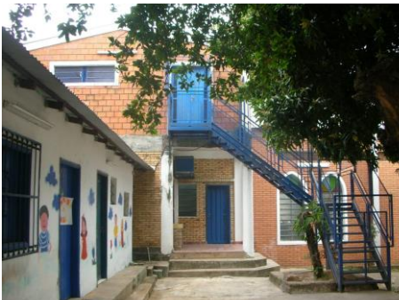
2010 upper storey to extension with access stairway built.
