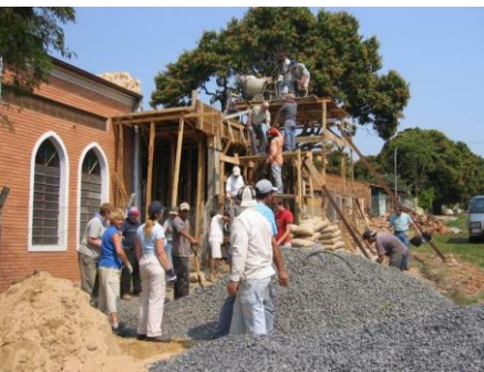
August 2005 team from churches in England concreting roof to extension.
