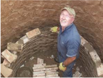
Building a well in 2010. Three more are to be funded in 2011.
