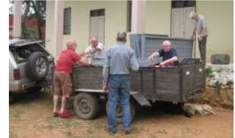
Loading new doors and windows for houses in Chaco
