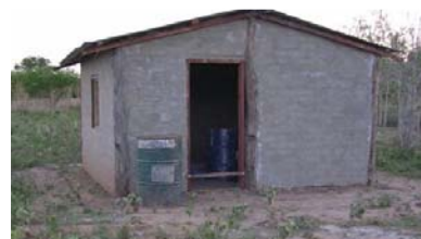
Adobe home under construction
