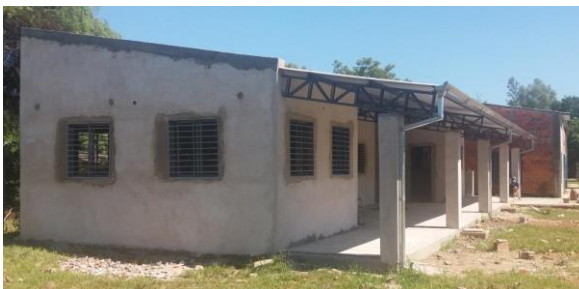
The new albergue at Remansito nearing completion in February 2017
