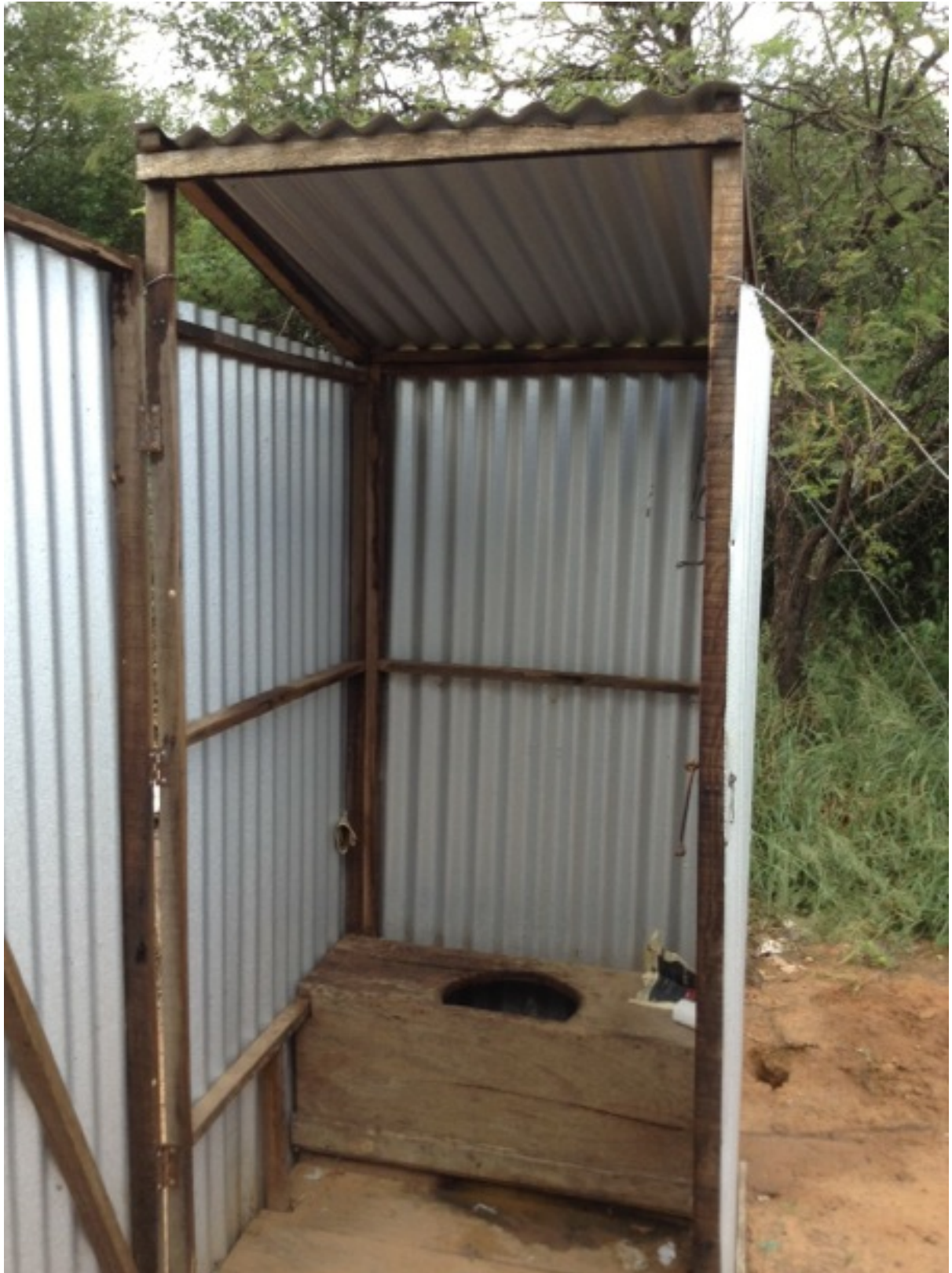
5. Typical latrine we have been making
