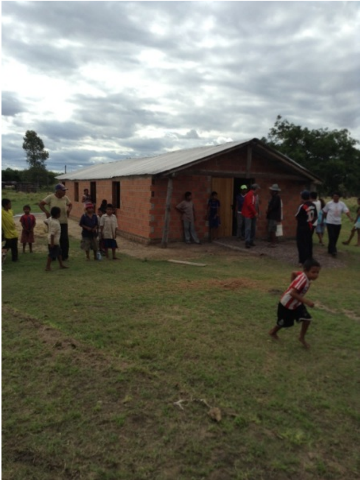
6. Colonia 24 Chapel. Original roof, new walls, doors, windows & floor
