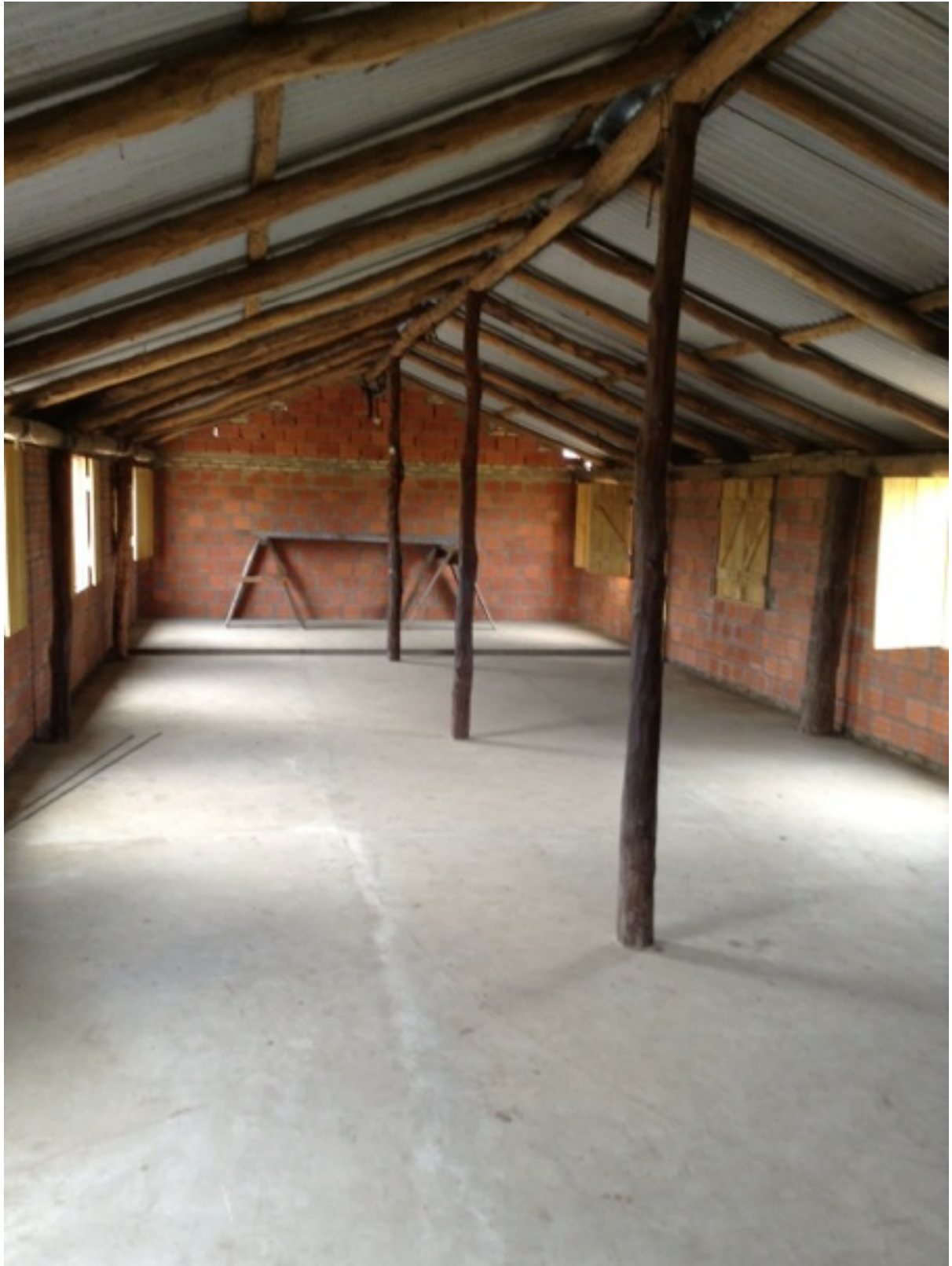
7. Colonia 24 Chapel. Original roof, new walls, doors, windows & floor
