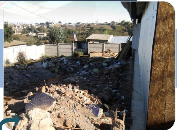
There used to be a church here. Now it is just rubble.
