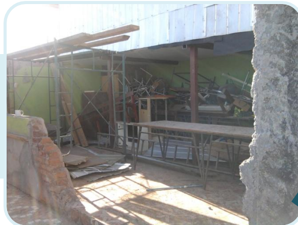
Feeding centre for children completely destroyed by the
