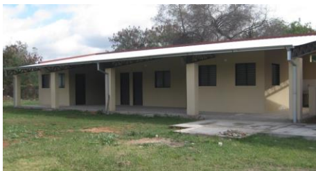
New albergue at Remansito nearing completion
