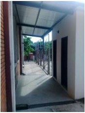
New toilet block at Zeballos Cue church
